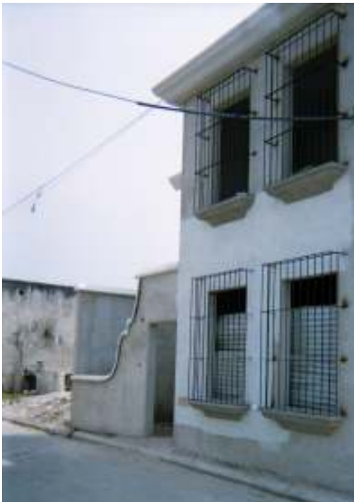
The Safe House- near completion
